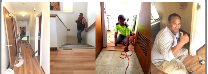
Puli Construction workers begin installing the floor boards.
