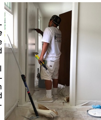
*Painting the interior of the convent.
