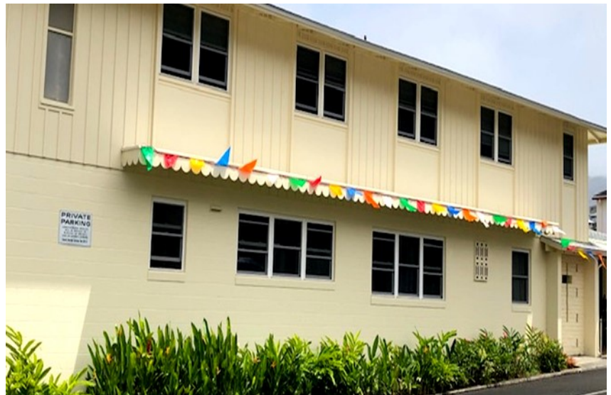
(Photos A & B) The former Religious Sisters' convent will be blessed and inaugurated as the new Pastoral Center this Sunday.
