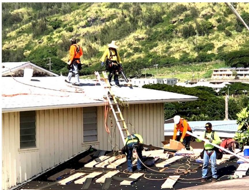
Photo 1: Re-roofing of the convent after 57 years.
