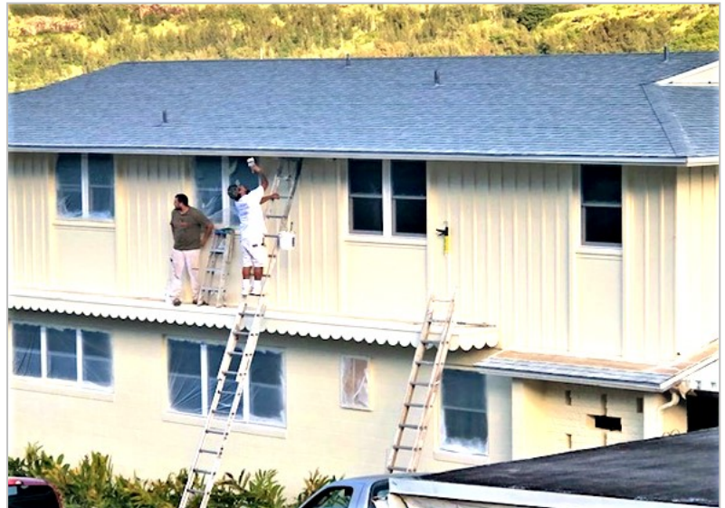
Photo 3: Repainting the Convent.
