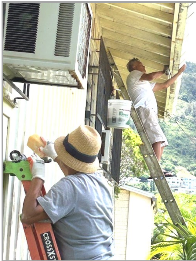
(Left Photo): SK Vicente Velasco & SK Renato dela Rosa prepping the rectory sides and awning for repainting by caulking and dusting off the molds, grimes and peeled off old paint.
