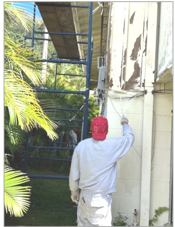
*CAULKING & REMOVING OF GRIMES, DUST, PEELED-OFF PAINTS & MOLDS
