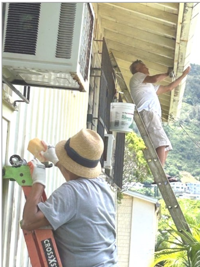
*CAULKING & REMOVING OF GRIMES, DUST, PEELED-OFF PAINTS & MOLDS
