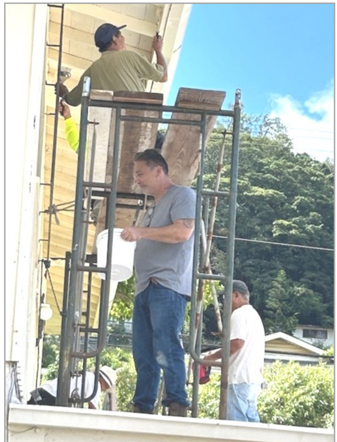
*CAULKING & REMOVING OF GRIMES, DUST, PEELED-OFF PAINTS & MOLDS
