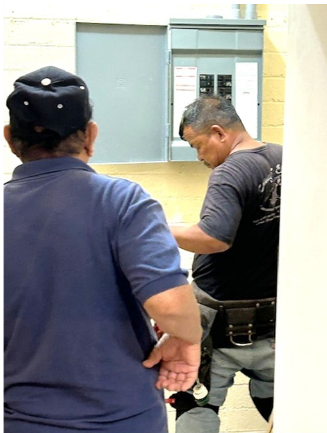
(Left & right photos): Remar Aquino put up a new switchboard panel for the A/C Units. The former switchboard serves as junction box.
