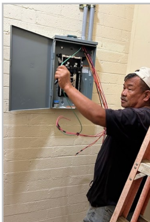
Remar Aquino installing the new panel board.
