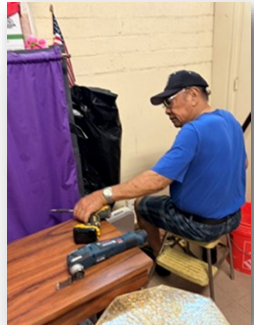
(Above photo): Roger Isidro fixing the crucifix stand at the sanctuary workroom.
